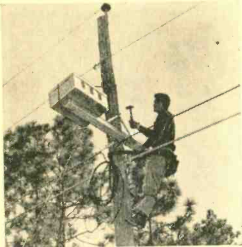
Signals from antennas feed trunk line which is main coax cable into town. Amplifiers are mounted on poles to boost distribution lines.
